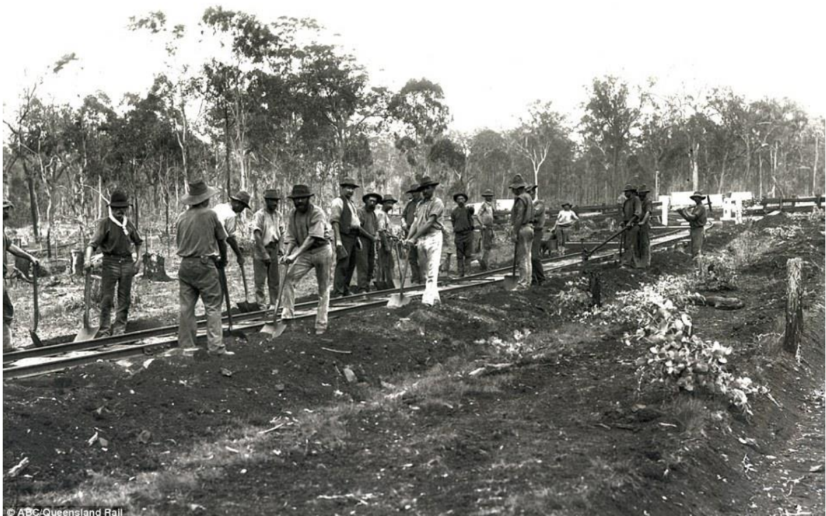
Railway workers building The Southern and Western Railway. Image Source: ABC/Queensland Rail
